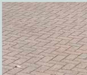
Herringbone brick paving
