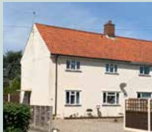
Pitched roof with red pantiles
