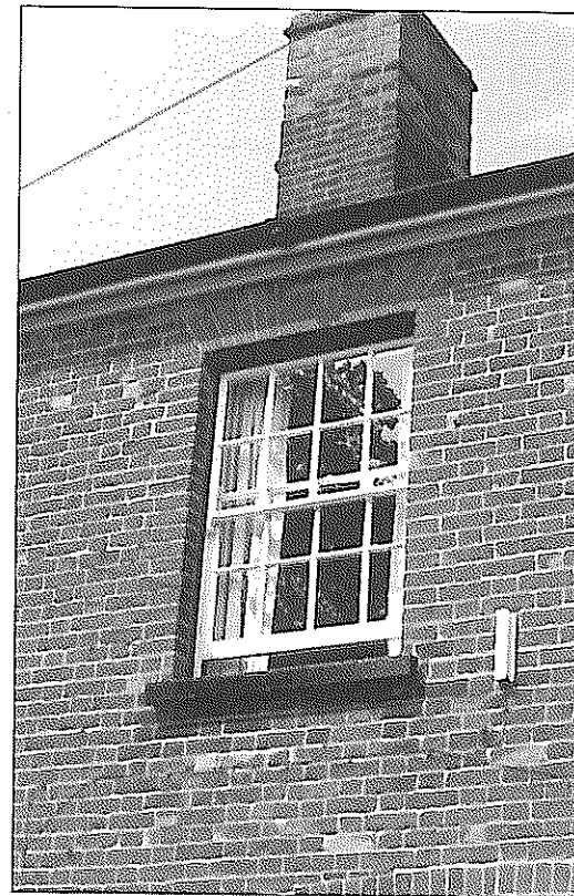
The traditional small-paned sash window.
