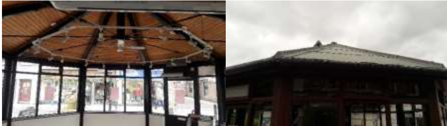
Figure 5: Timber Clad roof within the Octagon and Bitumen Type Exterior
