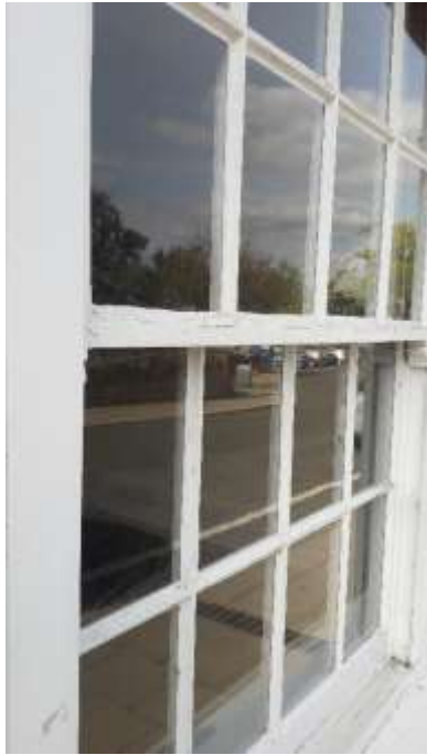
Figure 4: Single Glazed Wood Sash Windows to the Front of the Building
