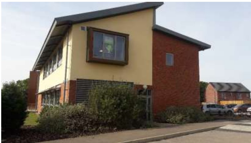
Figure 2: Side Elevation showing vented HVAC plant room
