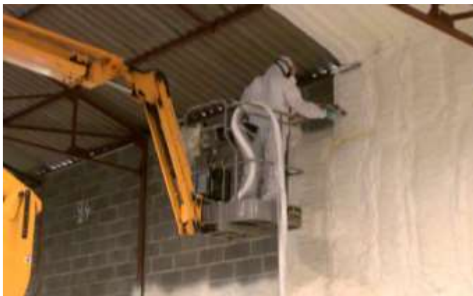
Figure 8: Spray Insulation
