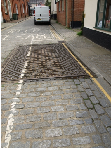
Figure 31: Cast iron cart weighbridge in the carriageway of Exchange Street.
