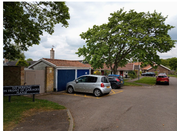
Garage with pantile roof
