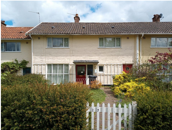
House on Windmill Green (North side)
