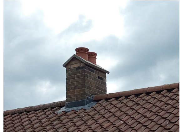
Characteristic chimney stacks
