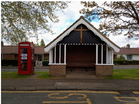
K6 telephone box and bus shelter Dating from 2000
