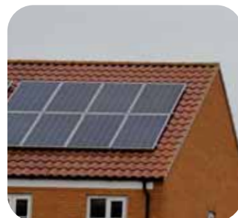
Clay tile and poorly integrated solar panel
