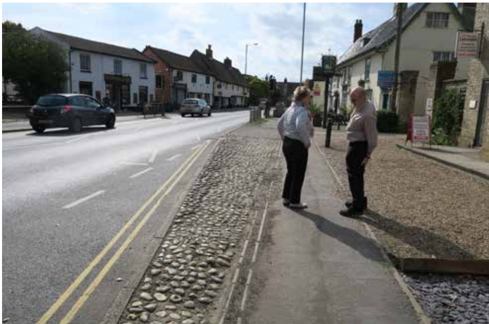
Fig. 3.1.2 Effective footway width reduced by areas of pebbled surface
