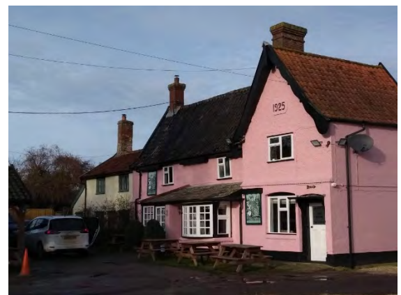
Pastel colour render, steep pitched roof and later C19th bargeboards at the Crown
