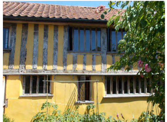
Stud timber framing and render Church Hill Farm Cottages
