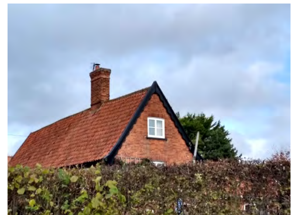
Steep gables, pantiles, red brick and bargeboards
