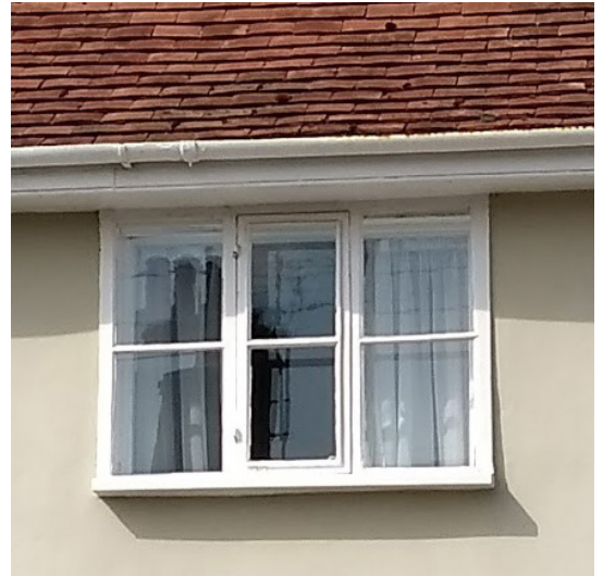
Original metal casements should be kept.
