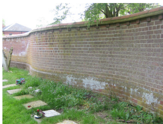
Crinkle crankle wall at the east boundary of The Old Rectory
