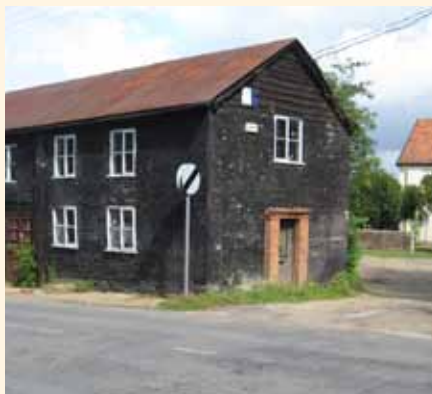
The Old Blue Warehouse
