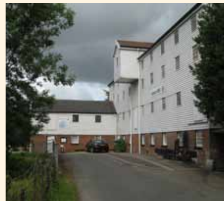
South side of the Mill
