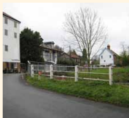
Railings just before the bridge at the south side of the Mill
