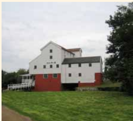
View of the Mill from the entrance drive
