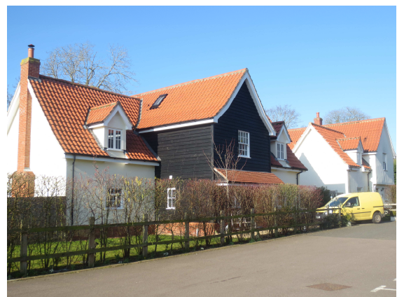
New housing built in a traditional scale using traditional render and black weatherboarding
