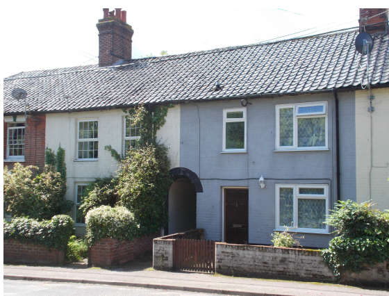
Varying replacement windows at Church Terrace
