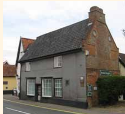
Old Manor House
