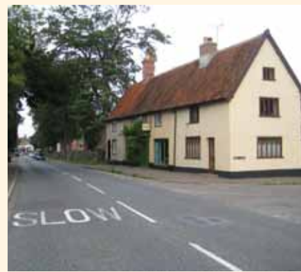
Junction north from Hall Lane
