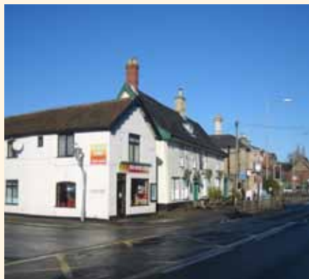
View of The Street at the Swan Lane junction
