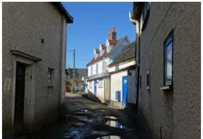
Potholed entrance to Old Post Office Yard
