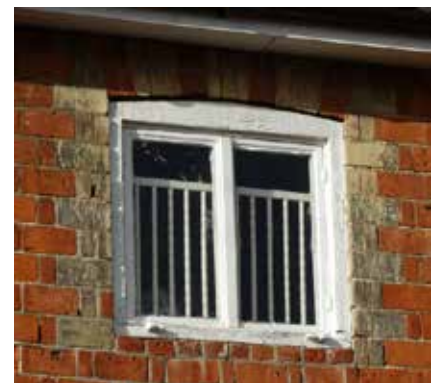
Gault brick is often used for detailing on simpler C19 houses and commercial buildings (This warehouse building also has an unusual rat trap brick bond)
