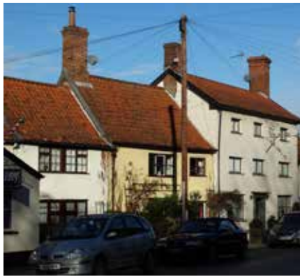
Rendered timber framing in Broad Street
