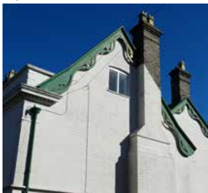
Decorative bargeboards are common
