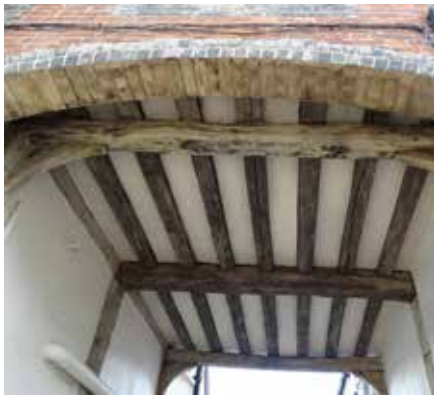
Brick refronting to timber framed house in Shipps Close
