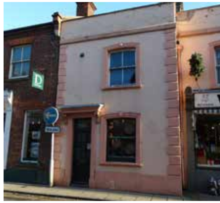
'Mock stone' plastered quoins and parapet hiding roof
