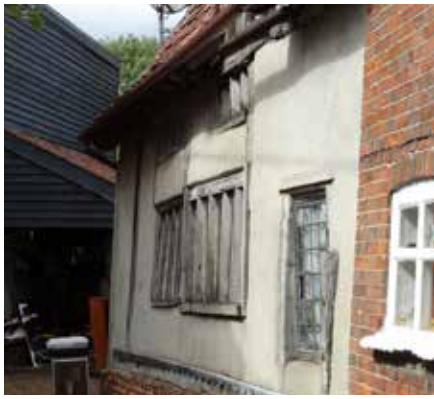
Post-medieval mullion windows
