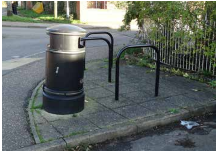
Poorly positioned cycle racks and bin
