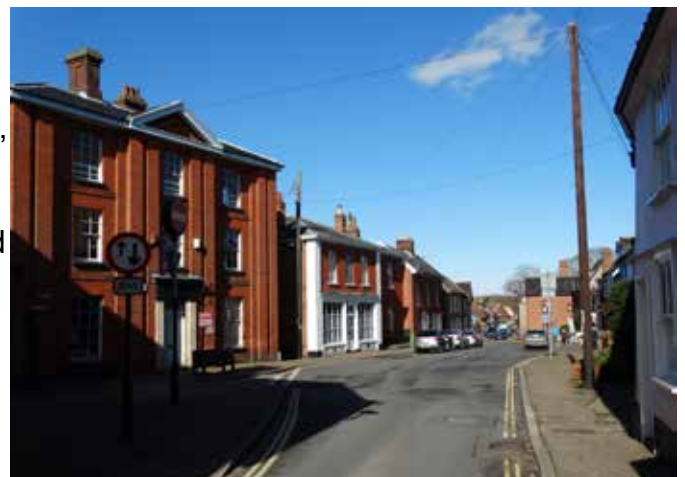
South end of Old Market Place looking north
