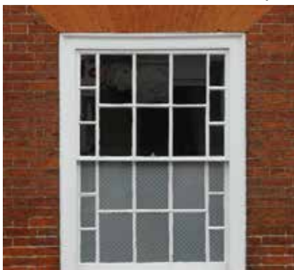
High quality georgian brick work and sash windows.
