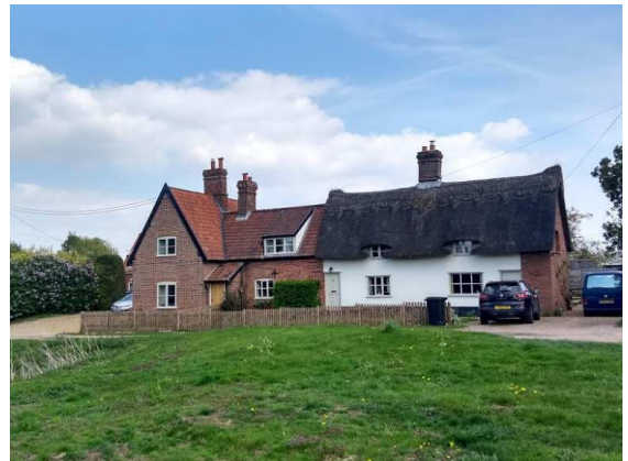
Render and thatch at Sunnyside and later extensions in brick and pantiles to adjoining north end.
