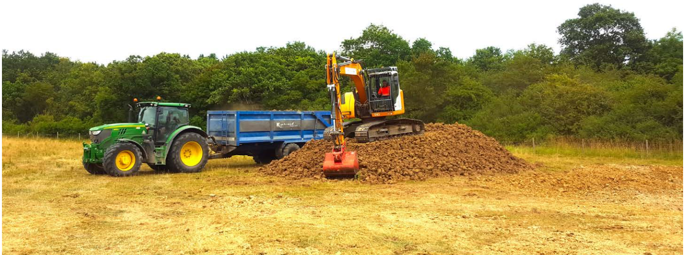
(c) Medium sized ponds of 200-500 m 2 can be excavated using 15 tonne machines. Larger ponds are more efficiently created with larger machines.
