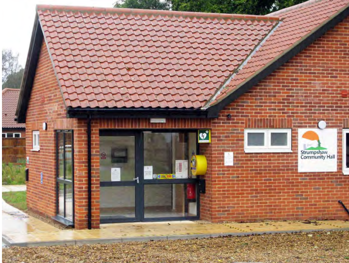
Figure 48: Strumpshaw Community Hall.
