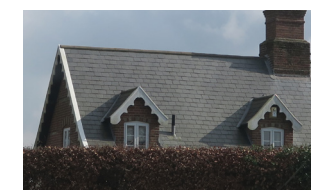
Figure 24: Dormers, white ornamental fascia board
