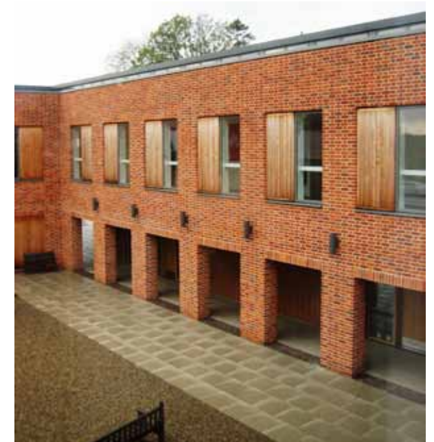
Langley School : New classroom building
