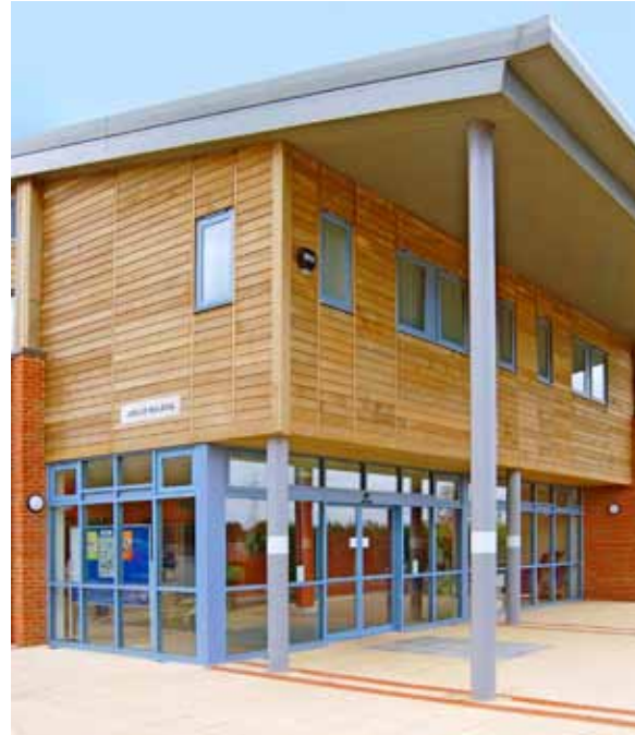
Easton College : Jubilee Building
