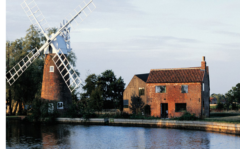
An innovative approach to the architecture of this extension to Hunsett Mill, Stalham, using asymmetric gabled forms, black charred timber and flush glazing to contrast with the restored mill and millkeepers cottage.
