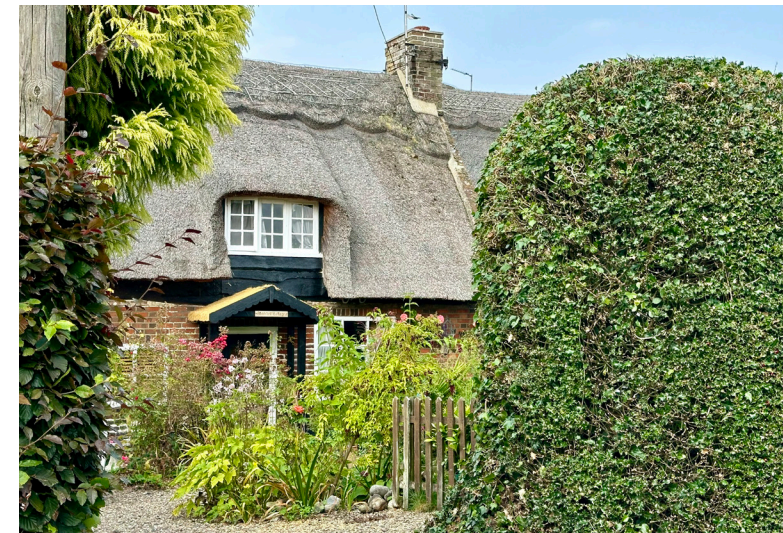
Thatched roofing, Blofield.
