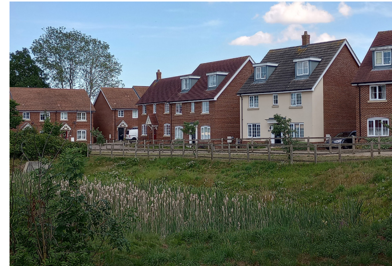
Attenuation basins balance flood resilience functions, and amenity value for residents, St Giles Park, Cringleford.
