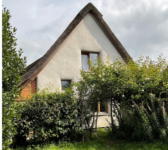
A highly sustainable thatched cottage in Hickling, built in straw bales, correctly using traditional forms and details.
