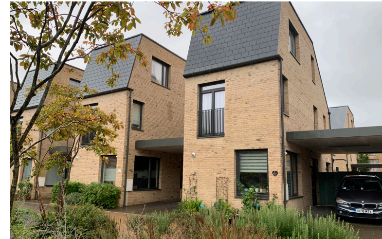
This development integrates car ports between a townhouse house type, Barton Park, Oxford.
