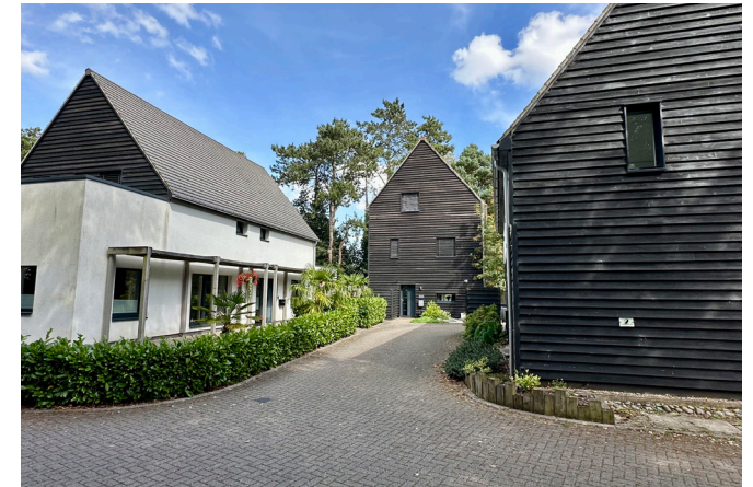
A shallow-plan form and steep roof pitch references traditional housing. Building orientation allows for solar gain in winter, with shading features to prevent overheating in summer. Carrowbreck, Norfolk.
