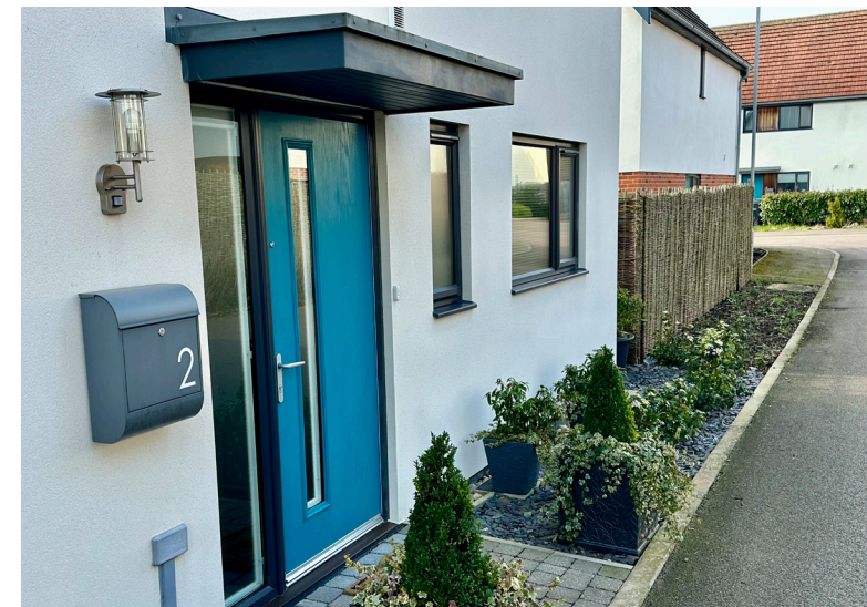
A simple modern porch with a coloured front door creates a welcoming entrance with space for residents to personalise. Hingham, Norfolk.
