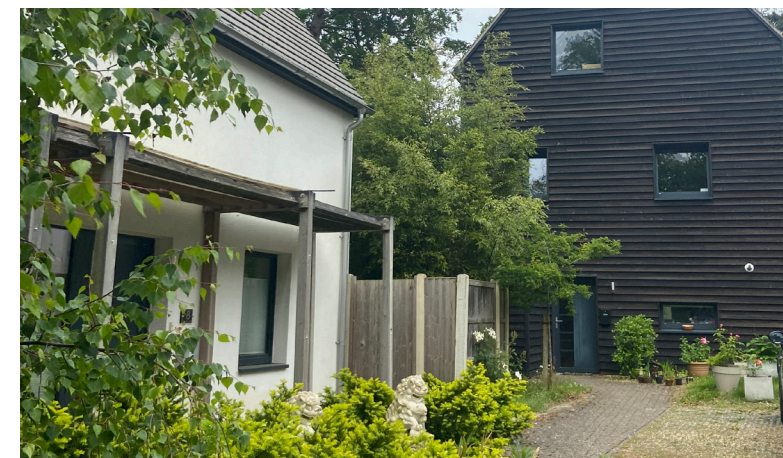
In this passivhaus development, close attention was paid to the use of materials. For example, specialised Porothersm blocks were used in the construction, which have thermal and acoustic efficiencies, and also use 95% less water than traditional.
