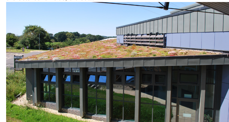
Green roof helps to integrate development into its countryside setting at Easton College, Norwich.
