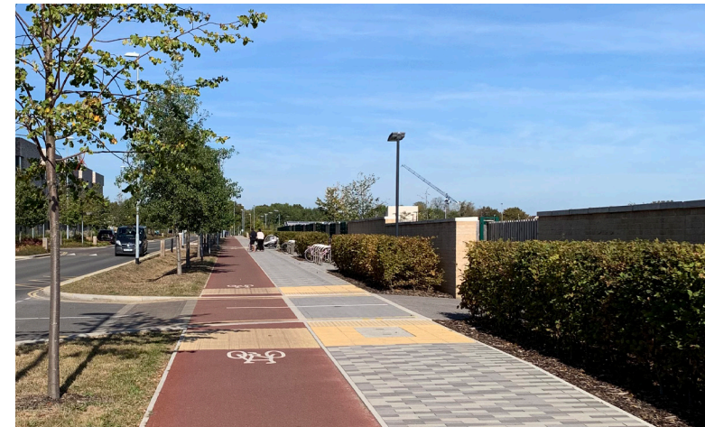
This primary street has segregated cycle lanes that respond to the importance of it as a main route within the movement hierarchy, in Eddington, Cambridge.
