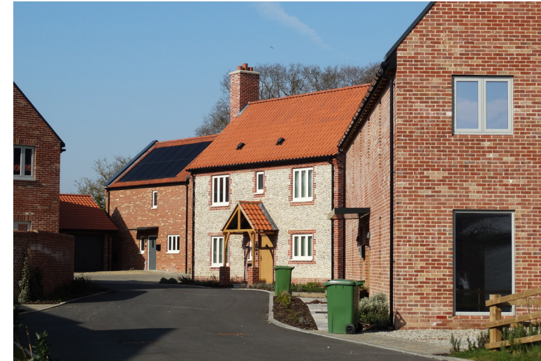
At this net carbon zero development in Northrepps, highly efficient design utilises triple-glazing, air source heat pumps and mechanical ventilation with heat recovery to minimise emissions and reduce energy consumption.
