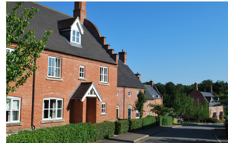
Coherent materials, strong landscaping, and articulate detailing creates a successful streetscene in this example in Trowse Newton.
