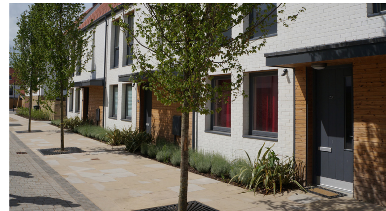
A modern interpretation of a terrace set close to the street at Derwenthorpe, York, with well-sized openings, vertically proportioned and with a planted privacy strip to overlook the public realm without loss of privacy, suitable for urban character.
