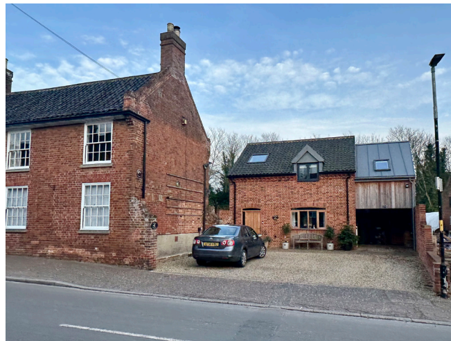
Use of brick for the main part of this infill development in Loddon, with its scale reduced by setting back part of the elevation and cladding it in different materials - timber and standing seam metal roofing.
