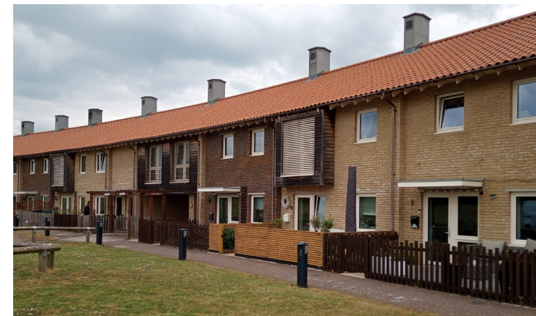
This terraced typology achieves Passivhaus standards, and has been sensitively integrated into a conservation area, adjacent to Taylor and Green Grade II Listed buildings, in Ditchingham.
