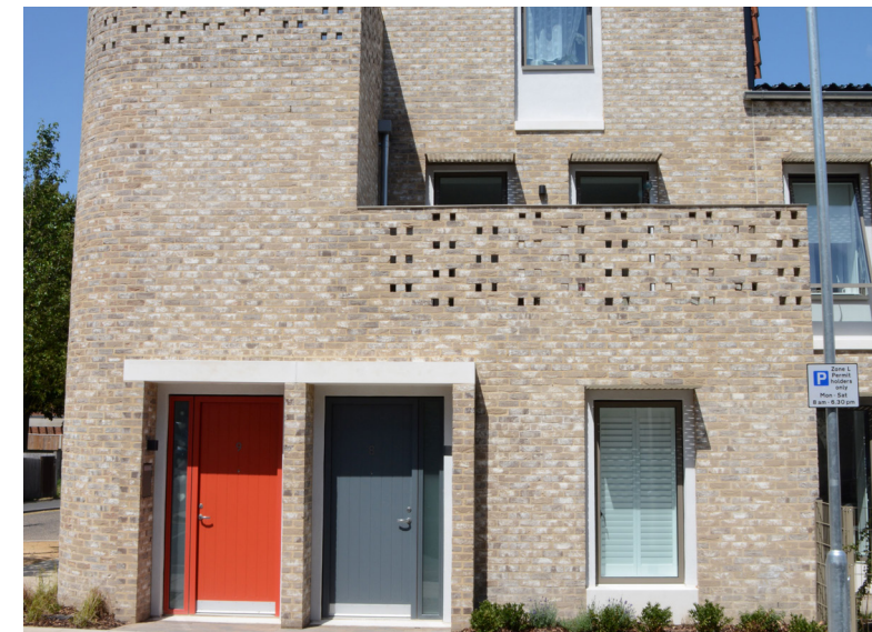
The location of this balcony and terrace have been arranged to protect residential privacy. Goldsmith Street in Norwich.
