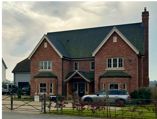
A generous porch at the entrance to this house in Pulham Market, also with well-detailed gables and chimney.
