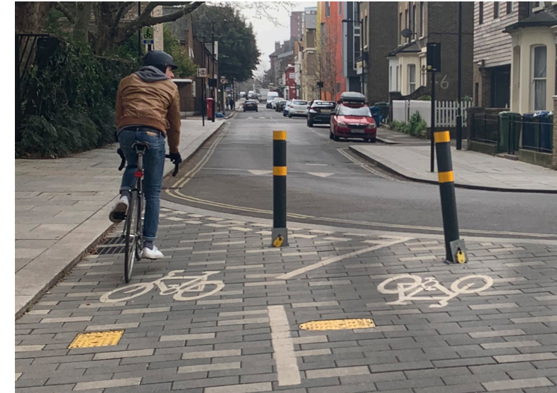
Modal filters allow cyclists to take the most direct route, in Southwark, London.
