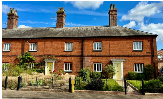
Generous front gardens set development back from the street edge, but a consistent and continuous building line retains a more urban character suited to Main Towns and Key Service Centres or the Norwich Fringe Settlements. Old Catton.
