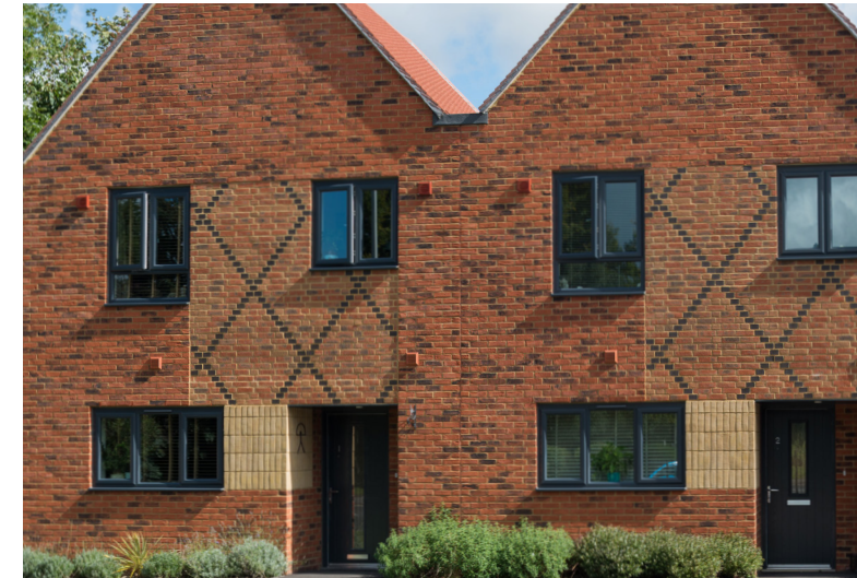
Brick diapering in Horsted Park, Chatham. This brick detailing improves character in a simple yet effective manner.
