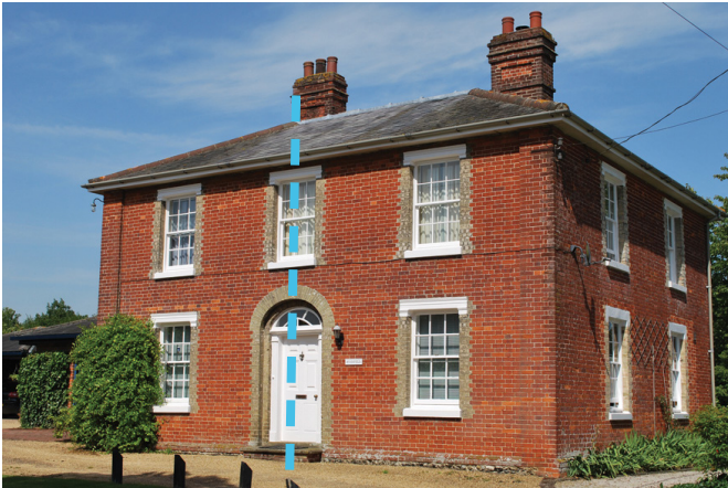
Well-balanced wide-fronted building form, hipped roof and elevation. Formal symmetry was often used to emphasise the status of important buildings including large homes, found in all area-types. Winfarthing, Diss
