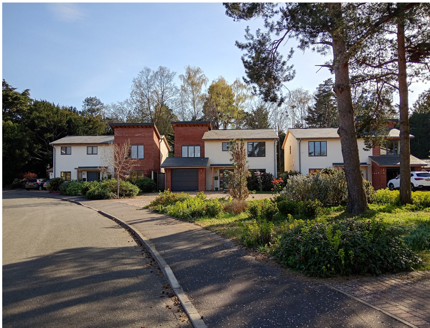
Development is shaped around existing established trees in Old Catton.
