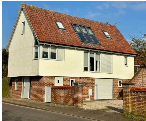
A contemporary interpretation of a jettied timber frame house in Wymondham, using elements of traditional timber frame houses together with modern well-proportioned openings, suitable for semi-rural or rural character.
