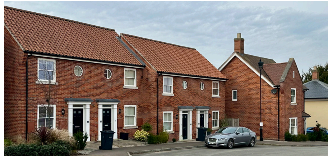
This variation in building line creates a positive widening of the street space that also allows for on-street parking spaces, in Trowse.
