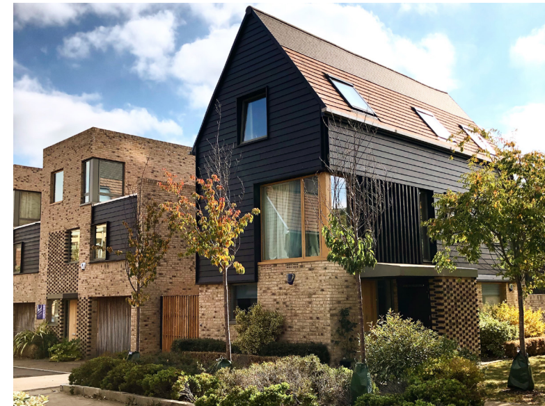
In this case, a change in built form, and additional height, marks this prominent corner at Great Kneighton in Cambridge.
