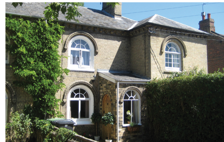
Costessey 'white' bricks were a locally-made traditional material, and contribute to the traditional vernacular and character of the town.
