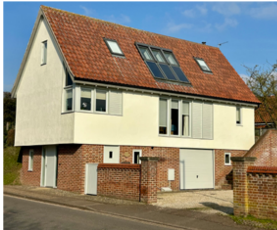
A contemporary interpretation of a jettied timber frame house in Wymondham, using elements of traditional timber frame houses together with modern well-proportioned openings, suitable for semi-rural or rural character.
