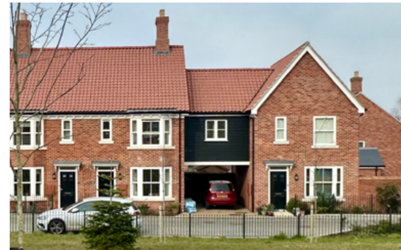
Car ports and integrated garages can be used positively in compact design solutions, in Trowse. These are likely to be most suitable in highly accessible locations.
