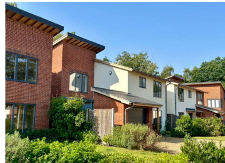
A varied roof form, with consistent materials and a consistent pitch used in a contemporary way, to create visual interest and a distinctive character at Parkside, Old Catton.
