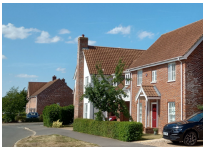
Home has good defensible space with an appropriate boundary treatment (a hedge in this case) which provides privacy for residents, but also some overlooking of the street, as seen here in Mulbarton.
