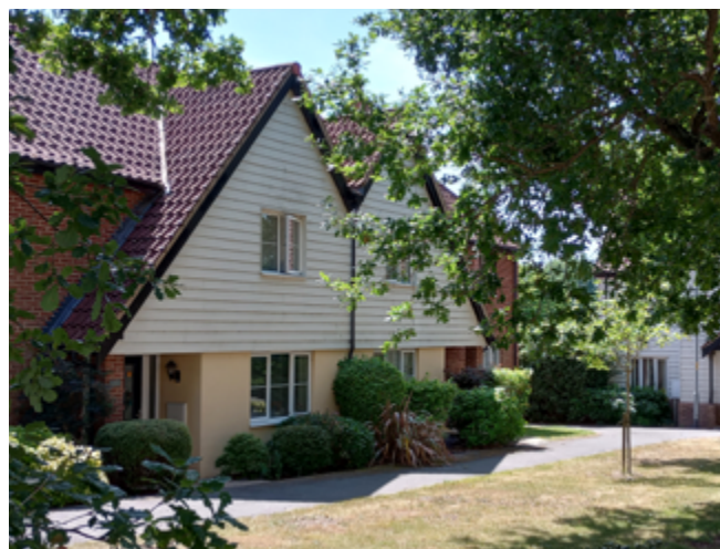
Even relatively narrow planted boundary treatments help create a buffer to the public realm, Poringland.
