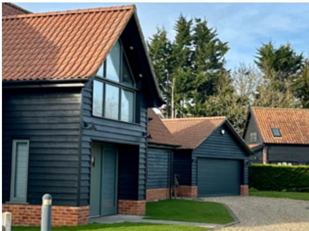
A generous entrance that provides shelter and is clearly marked by a wide recess that suits the rural or semi-rural character of these barn-like forms in Tacolneston.
