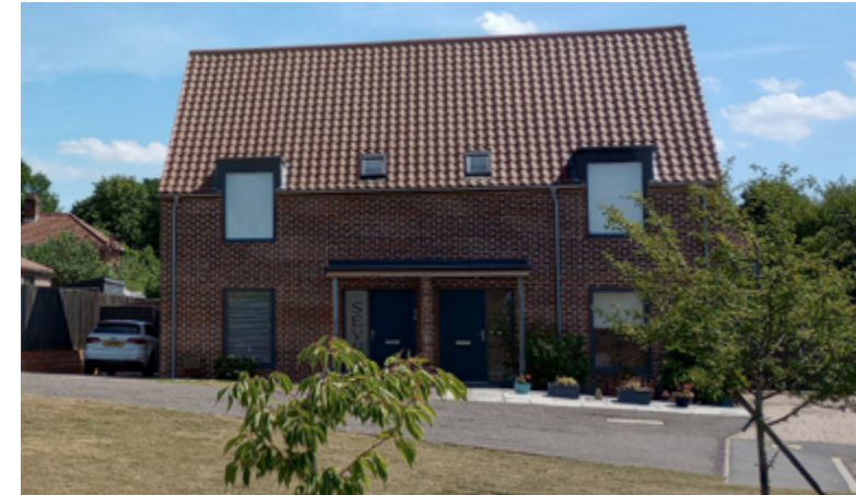
A combination of a porch, and bold signage help to mark this entrance in Stoke Holy Cross.
