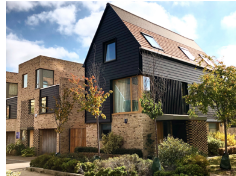
In this case, a change in built form, and additional height, marks this prominent corner at Great Kneighton in Cambridge.
