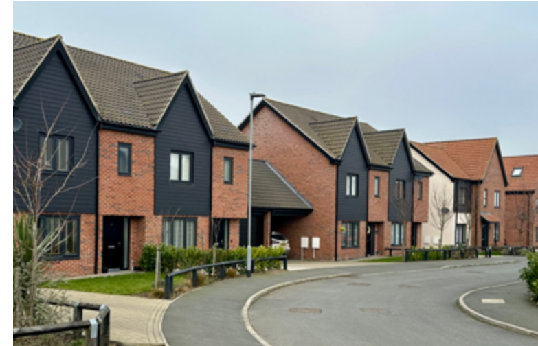
Cars are integrated behind the building line on this street in Harleston.
