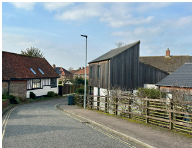
Roof form divided into two monopitches so that it fits into the scale of the townscape at Albansfield, Wymondham.
