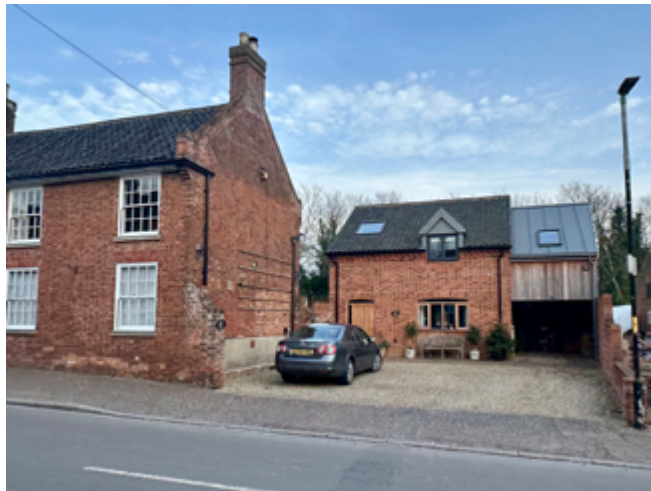
Use of brick for the main part of this infill development in Loddon, with its scale reduced by setting back part of the elevation and cladding it in different materials - timber and standing seam metal roofing.
