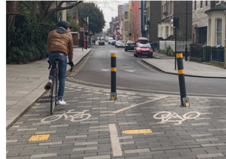
Modal filters allow cyclists to take the most direct route, in Southwark, London.
