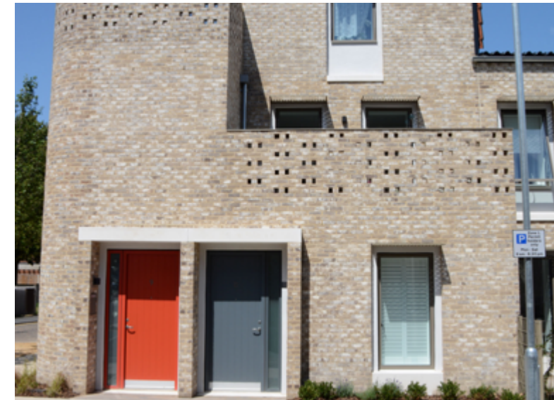
The location of this balcony and terrace have been arranged to protect residential privacy. Goldsmith Street in Norwich.
