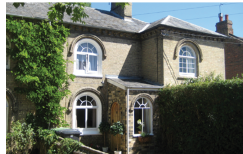
Costessey 'white' bricks were a locally-made traditional material, and contribute to the traditional vernacular and character of the town.
