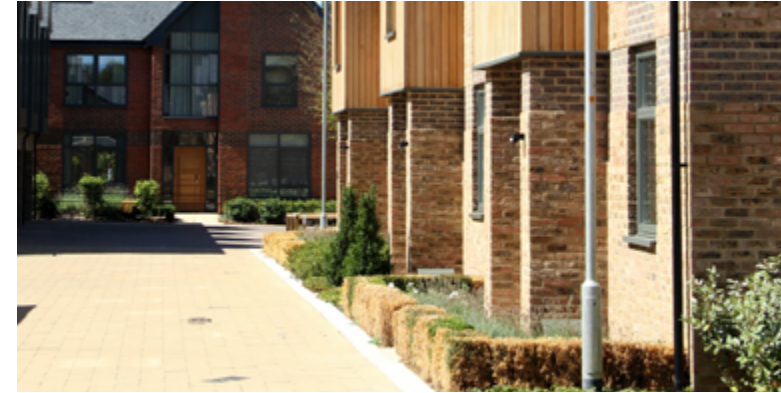
Defensible space at the front of these homes provides privacy for residents in Longcroft.
