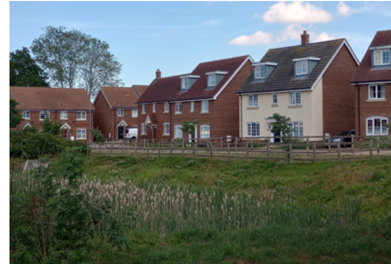
Attenuation basins balance flood resilience functions, and amenity value for residents, St Giles Park, Cringleford.
