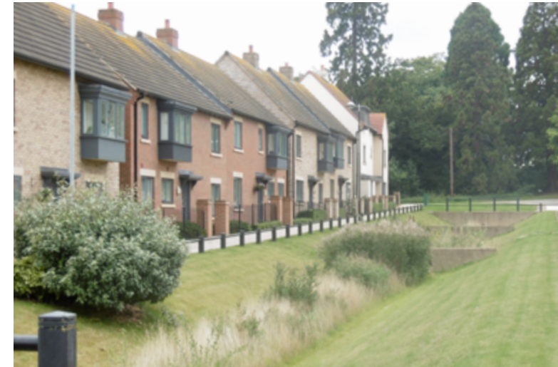
This space has been designed to make a feature of the flood management, with buildings orientated to overlook and frame the swale, in Northampton.
