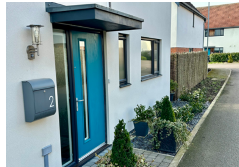
A simple modern porch with a coloured front door creates a welcoming entrance with space for residents to personalise. Hingham, Norfolk.
