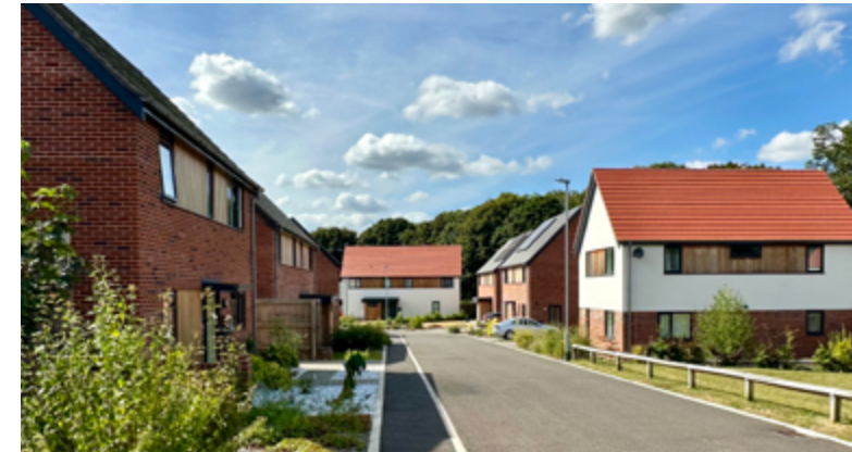
On-plot planting, and a consistent building line create a positive and defined street character in Taverham.
