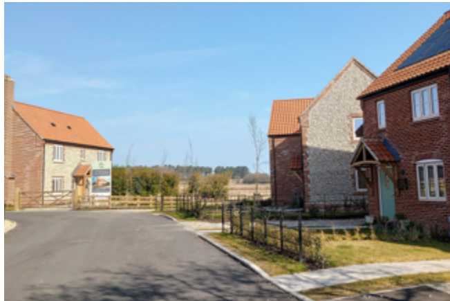
Houses are orientated around open spaces to create a soft and informal edge to this scheme in Northrepps.
