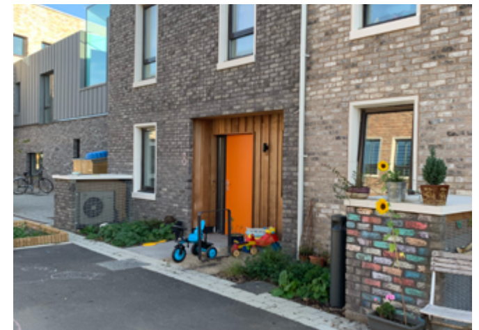
Heat pumps are carefully integrated in front of homes at this development on Marmalade Lane, Cambridge.
