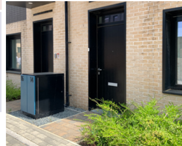
High quality solutions that provide secure storage for bins, and utility infrastructure that does not compromise the public realm or homeowner's private spaces.
