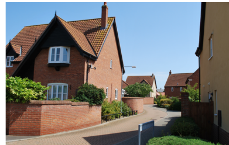
On this side return, windows overlook the street, with planting to provide some privacy, in Poringland.
