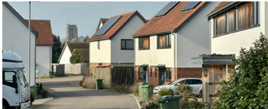
The built form and street layout preserves a view towards the church nearby, in Hingham.
