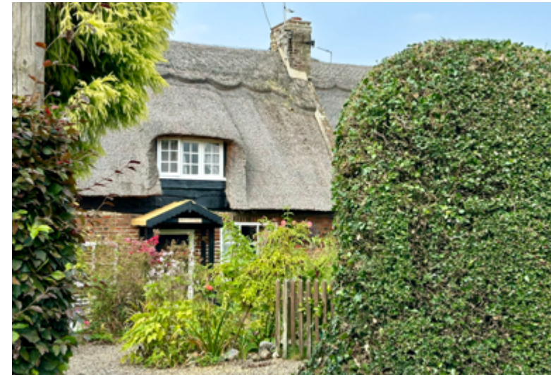
Thatched roofing, Blofield.
