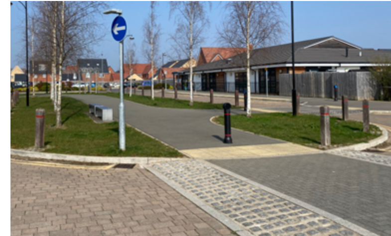
Raised table enables pedestrians, cyclists and wheelchair users to continue along a direct route the development in Biggleswade.
