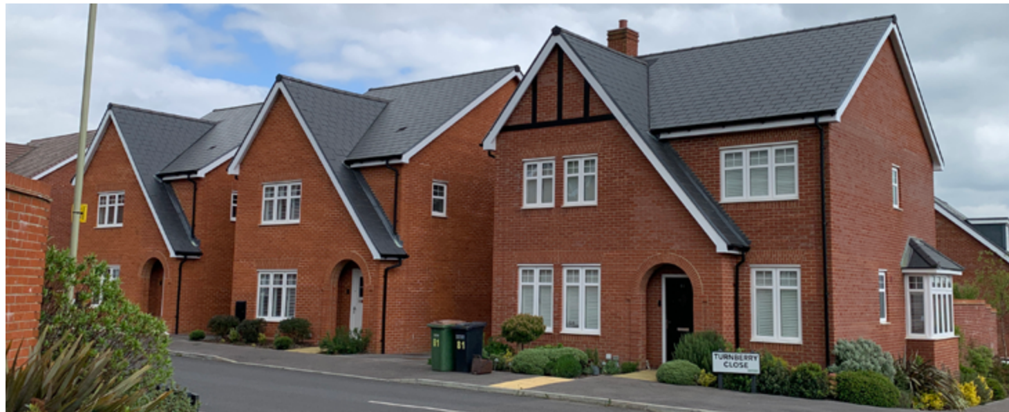
Roof form creates a regular rhythm which creates character along this street in Eastleigh.
