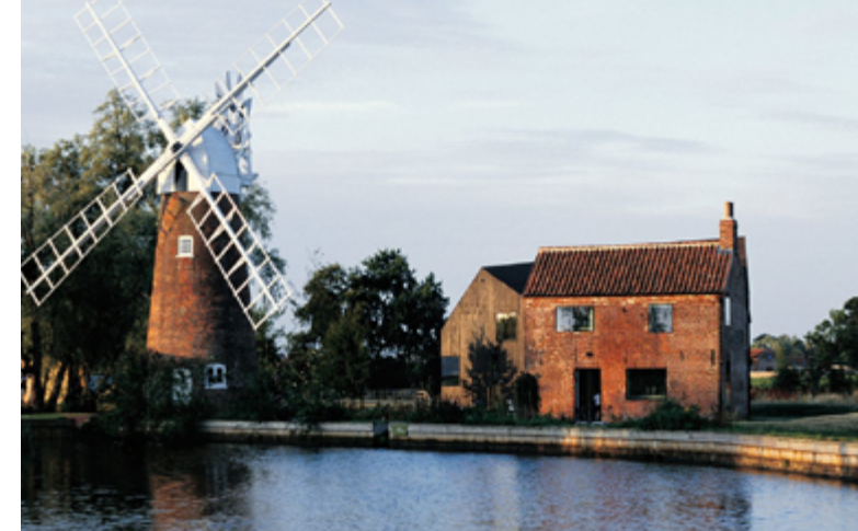
An innovative approach to the architecture of this extension to Hunsett Mill, Stalham, using asymmetric gabled forms, black charred timber and flush glazing to contrast with the restored mill and millkeepers cottage.
