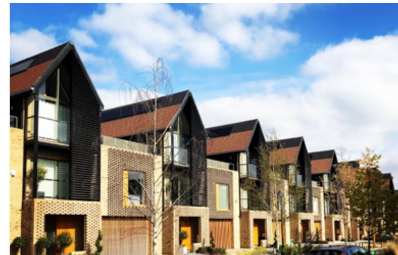
Well-proportioned roof forms with gable ends, and with solar panels integrated into the design at Great Kneighton, Cambridge.
