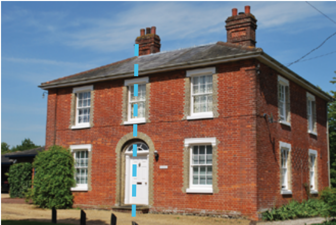
Well-balanced wide-fronted building form, hipped roof and elevation. Formal symmetry was often used to emphasise the status of important buildings including large homes, found in all area-types. Winfarthing, Diss
