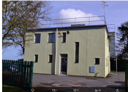
Left and right: The Control Tower, restored in 2006-7.
