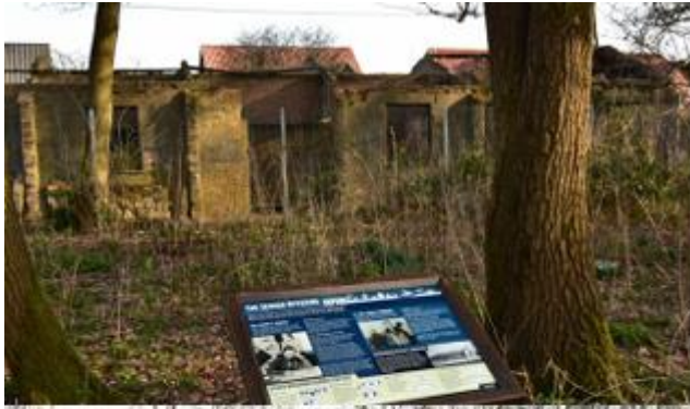
Top left: officers quarters, mess hall and communal canteen at Newman Woods
