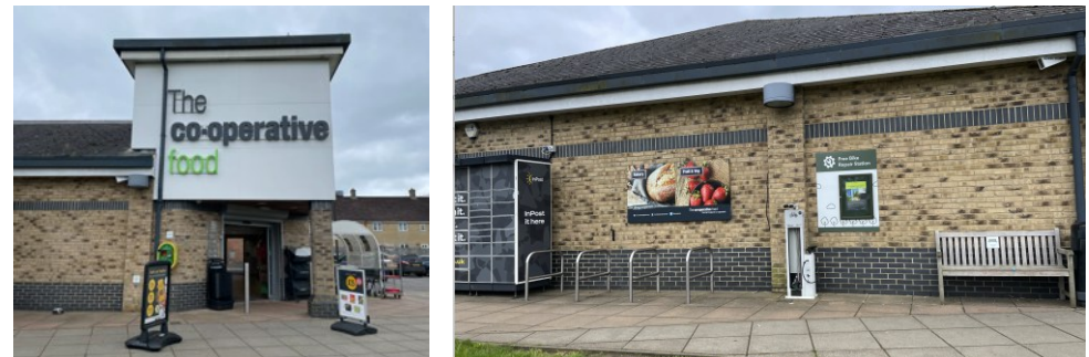
Figure 85: Medium sized supermarket possible for district centre, including parcel collection point and bike repair point. Co-op supermarket, Mulbarton, Norfolk. Source: own.
