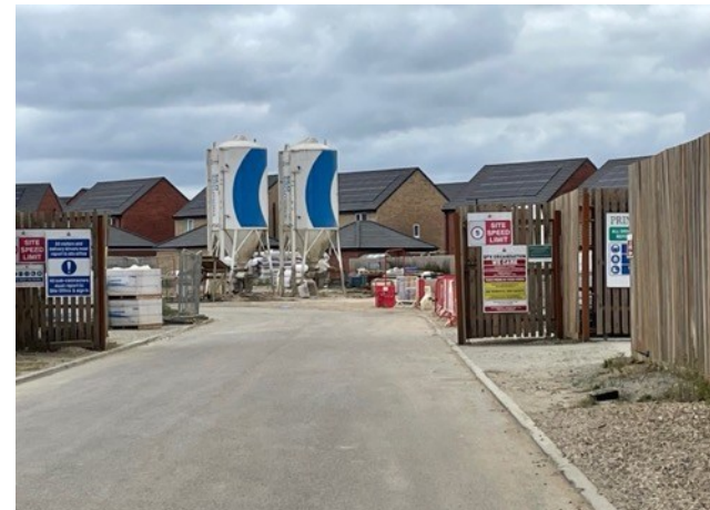
Figure 100: Solar panels incorporated into the roof. Green Lane West, Rackheath. Source:
