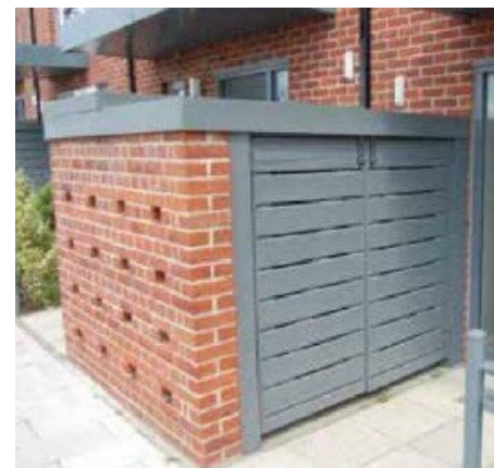
Figure 95: Incorporated bin storage. Centenary Quays, Southampton. Source: www.designbuildings.co.uk
