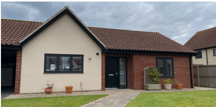
Figure 92: Accessible bungalow. Princes Park, Rackheath, Norfolk. Source: own.
