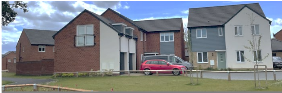
Figure 32: Varied roof heights and pitches. Princes Park estate, Rackheath, Norfolk. Source: own.
