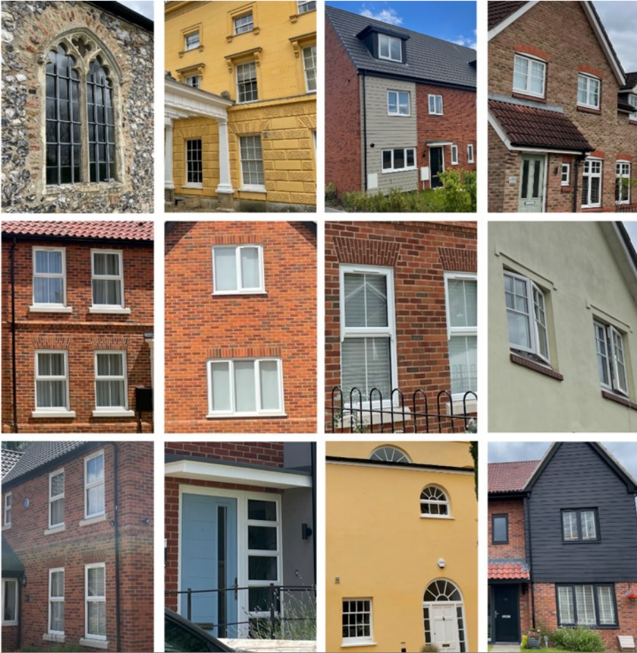
Figure 31: A variety of Rackheath quality windows, gives character and interest to the streetscape. Common types include mock sash windows, single and double hung windows, casement windows, shaped windows. Source: own.
