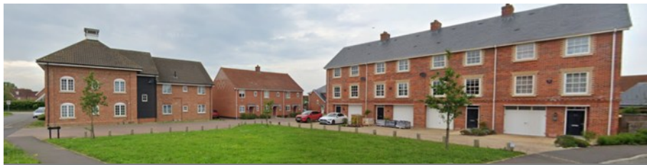
Figure 33: Varied roof heights and pitches. Mulbarton, Norfolk. Source: Google Maps, Street View.
