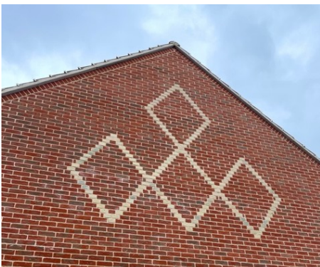
Figure 29: Diapering, brick detailing adds interest to an otherwise blank wall. Mulbarton, Norfolk. Source: own.
