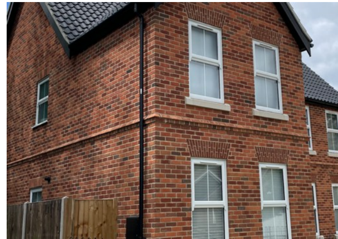
Figure 26: Architectural detailing on properties add interest and break up the facade. The Landings estate, Rackheath, Norfolk. Source: own.
