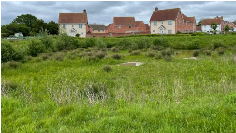
Figure 65: Wetland SuDS, providing a green entrance to the development. Mulbarton, Norfolk. Source: own.
