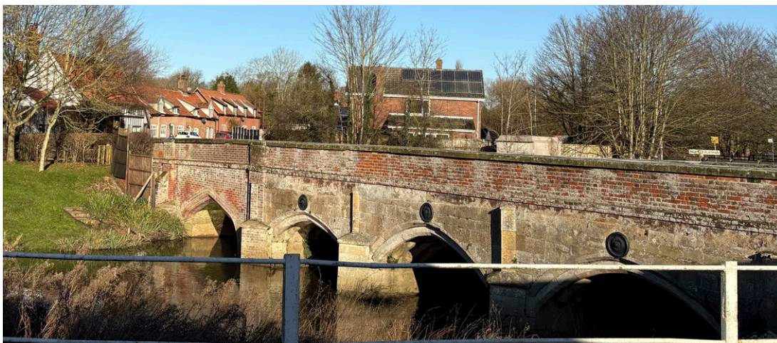
Figure 22: Newton Flotman Old Bridge.
