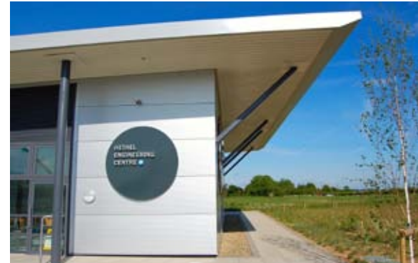
Left: Easton College Jubilee 3 Building. Top-left and top-right: Hethel Engineering Centre. Examples of buildings which use features such as roof overhangs and structural elements which not only create shading but also introduce three-dimensional modelling to the building façade
