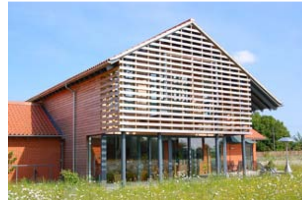
Dickleburgh: Example showing how solar shading has been successfully incorporated into the architectural design of the façade
