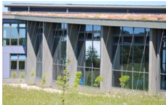
Left: Easton College Jubilee 3 Building. Top-left and top-right: Hethel Engineering Centre. Examples of buildings which use features such as roof overhangs and structural elements which not only create shading but also introduce three-dimensional modelling to the building façade
