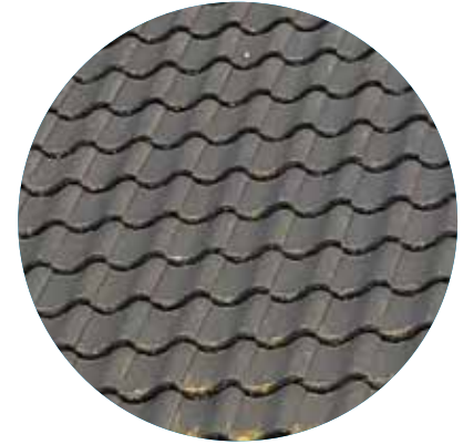
Black glazed pantile roof
