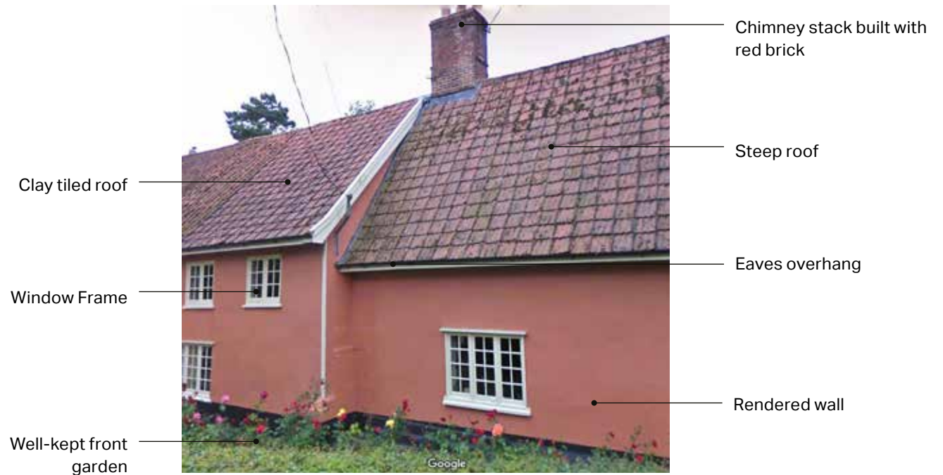
Figure 137: A detached residential house on Rectory Road.
