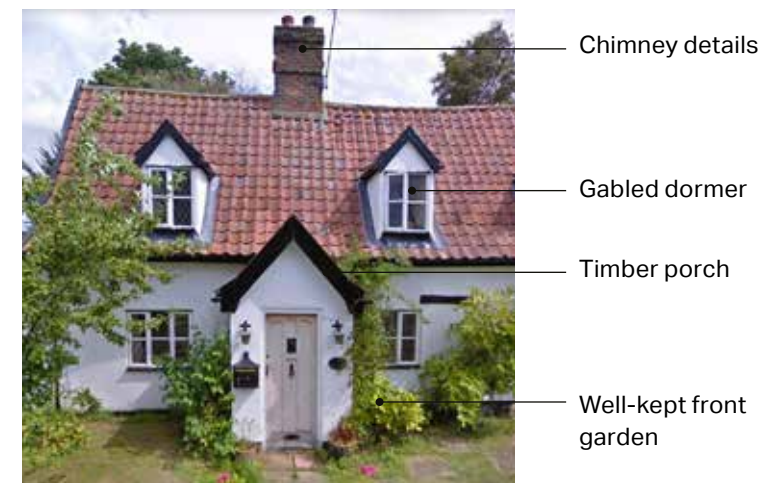
Figure 112: A family house on Hall Lane, Shimpling.
