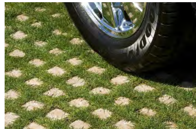
Figure 25: Permeable paving used for parking spaces.
