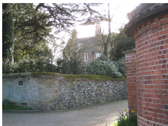
Wall to The Grange
