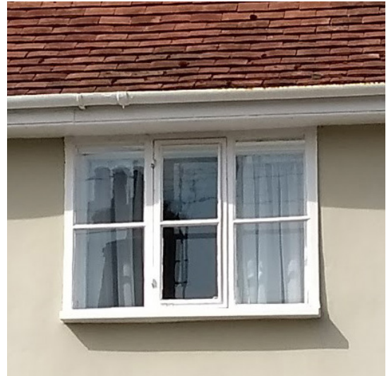
Original metal casements should be kept.
