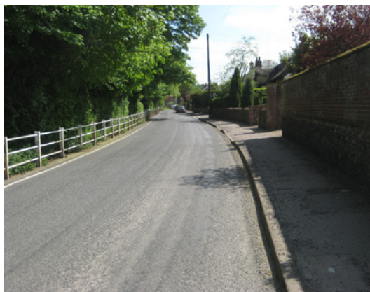
Looking South along The Street - railings & stream to the left side.
