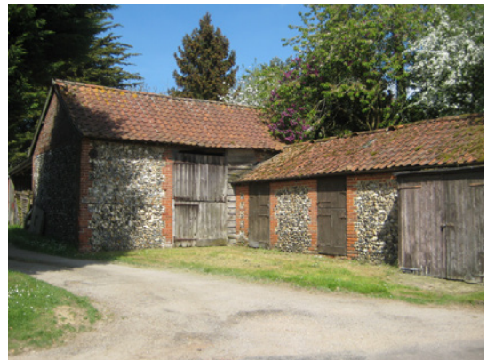
Flint outbuildings Cargate Lane
