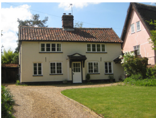
Nethergate Cottage, The Street
