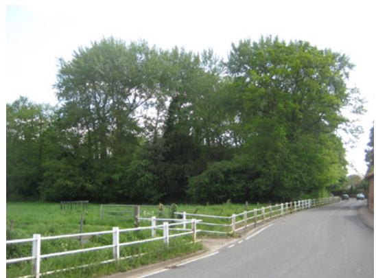
Railings at the boundary of the hedgerow along The Street
