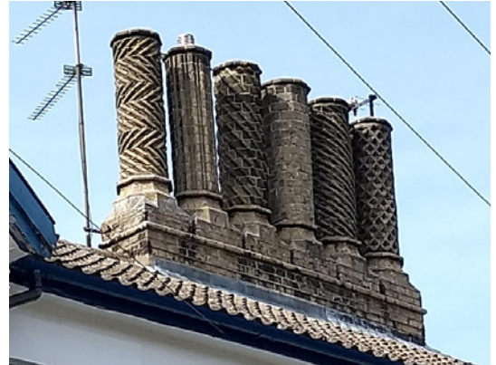
Chimney Stacks 39 - 45 The Street
