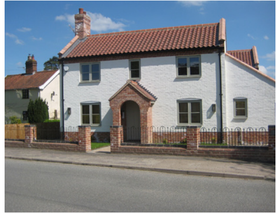
New traditional windows at White Cottage
