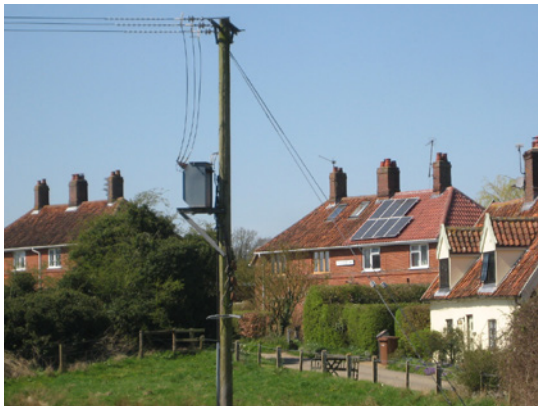
View split by telegraph pole
