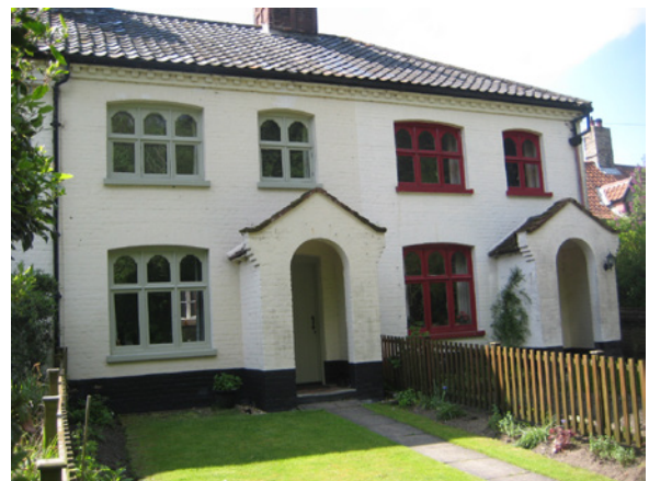
Gothic Windows at the New Cottages
