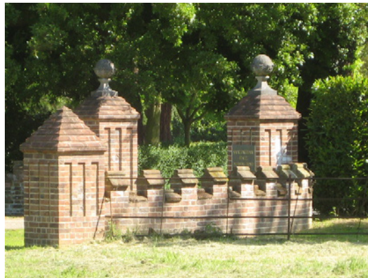
Wall and pillars at entrance to Saxlingham Hall.
