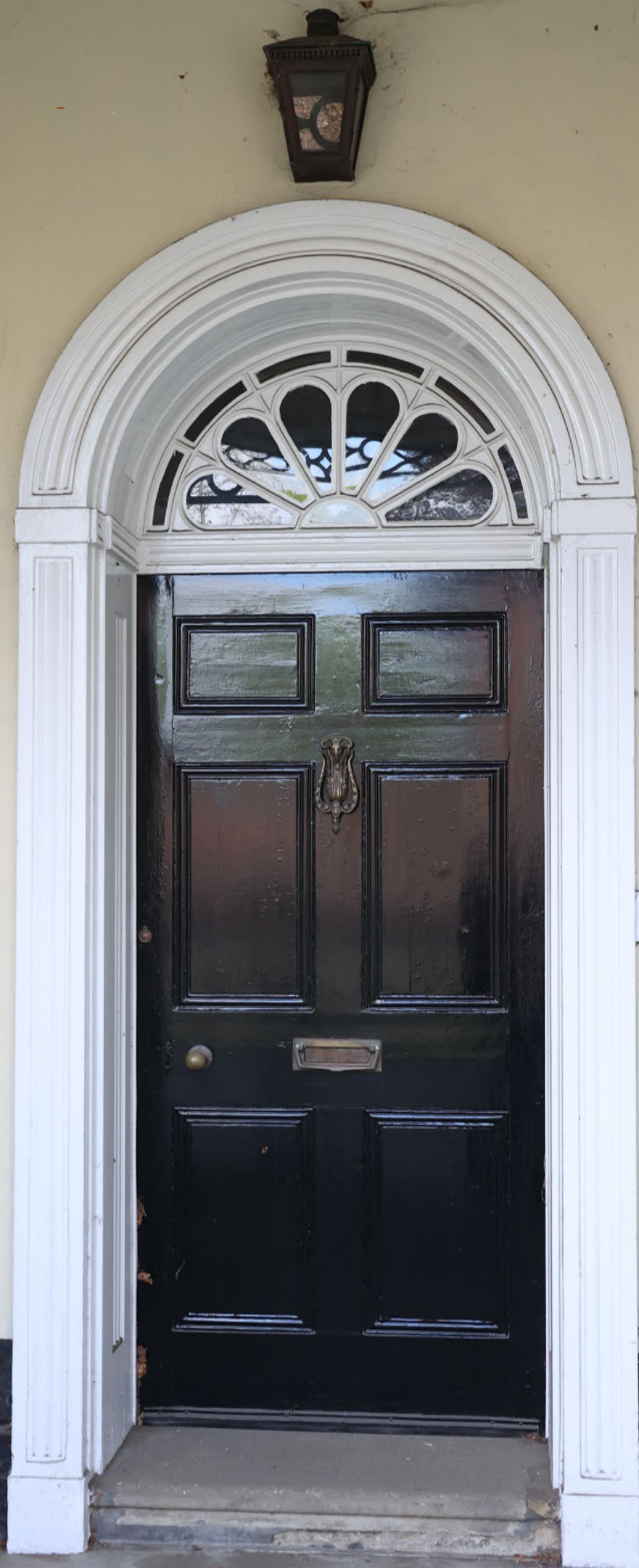
Figure 50: Georgian front door
