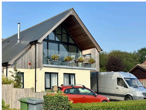
First floor living room with large south-facing windows to overlook the river in Reedham, set back with a deep roof overhang that provides solar shading in summer.
