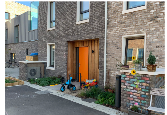
Heat pumps are carefully integrated in front of homes at this development on Marmalade Lane, Cambridge.
