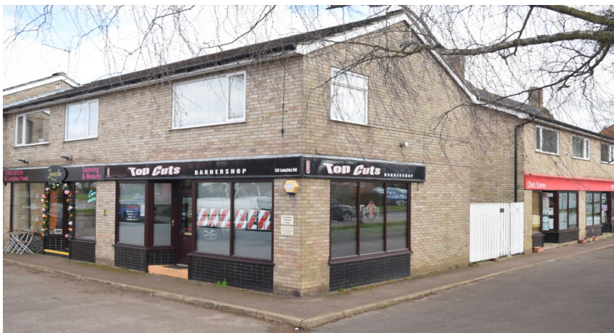
Photos of part of Chedgrave’s Shopping Strip
