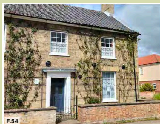
Figure 54: Photo of a 2 storey dwelling in Chedgrave.
