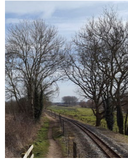
V. Bure Valley Path Pile Bridge to Little Hautbois
