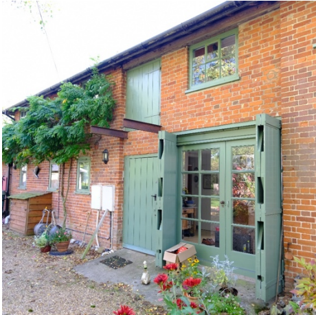
Rushall house, showing the original features of the threshing barn.
