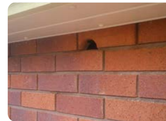
Figure 35: Example of a Swift brick under an eave.
