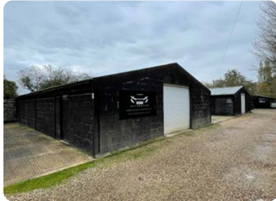
Figure 23: Units 3 and 4, Brick Kiln Lane.
