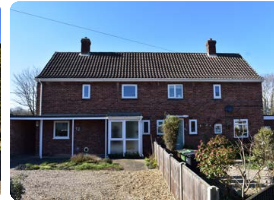
Figure 17: Housing at Station Close (CA3f).
