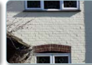
Light painted brick with brick lintel arches
