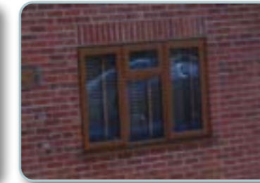
Timber casement windows with brick lintel
