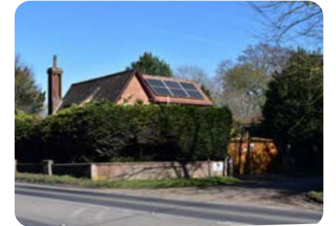
Figure 28: Example of residential dwelling setback further with hedges providing privacy.
