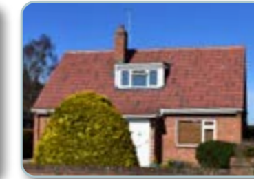
Gabled clay-tiled roof with shed dormer
