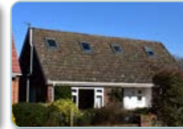
Gabled cement-pantiled roof with skylight
