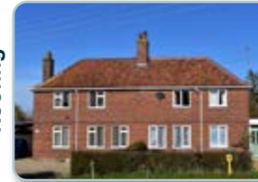
Hipped clay-tiled roof
