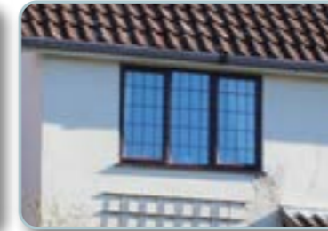
Flush 3-panel casement window with timber lintel
