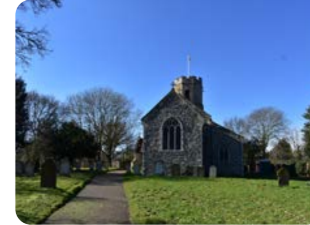
Figure 32: View of the church from eastern approach.
