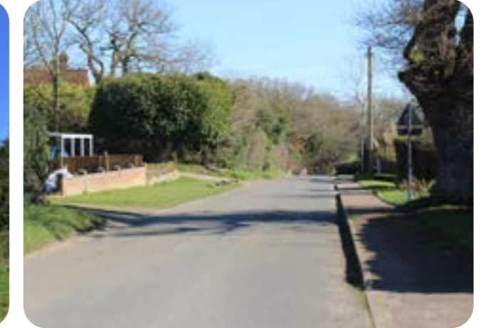
Figure 31: Views along Church Road towards the A140.
