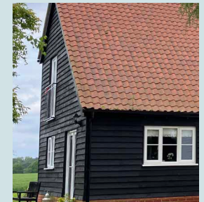
Timber weatherboarding
