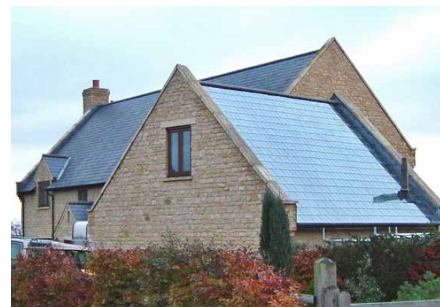
Figure 34: Positive example of implementing solar panels since the design stage.
