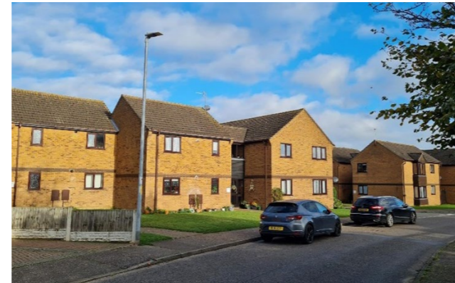
Figure 22: Flats within CA9: Cardington Court that shows the highly consistent building design within the area.
