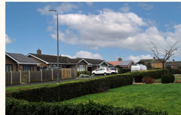
Figure 105: It is characteristic of neighbouring bungalows to be consistent in mass, material use, setback and orientation along a road.
