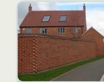
High hardscaped walls (brick, cement) without any breaks/openings
