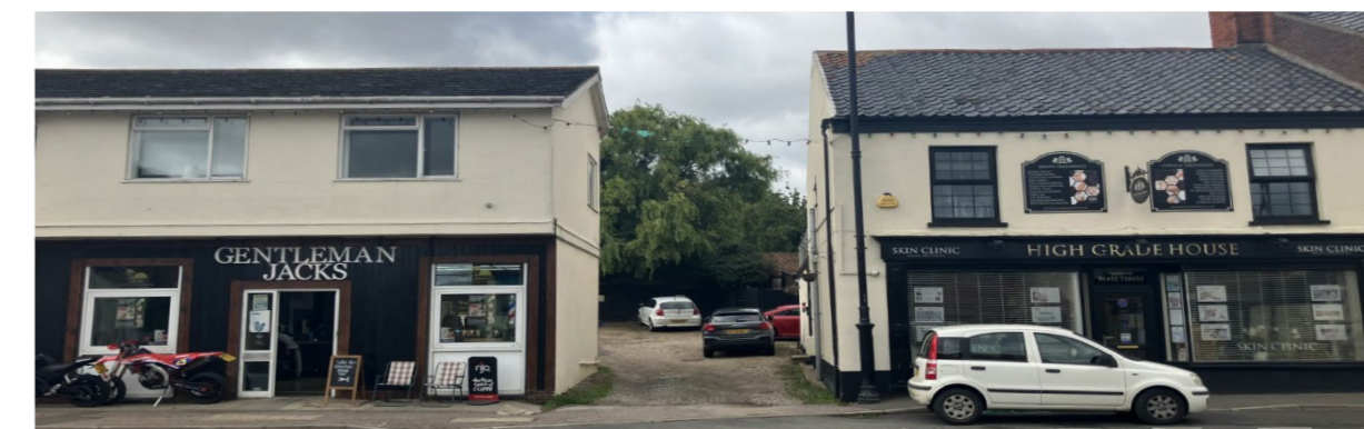
Figure 61: Positive example within Acle of well-designed shop fronts that integrate both traditional and contemporary qualities appropriate to the existing façade.
