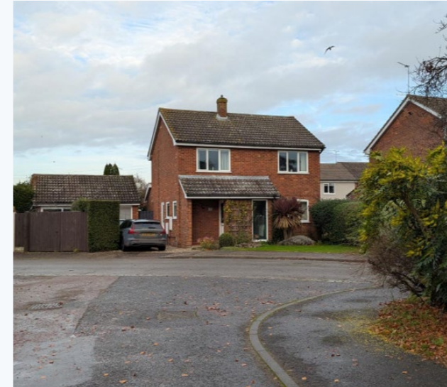
Figure 80: Most dwellings have on-plot parking and a front garden, which adds an open feel to a more dense area of the village.
