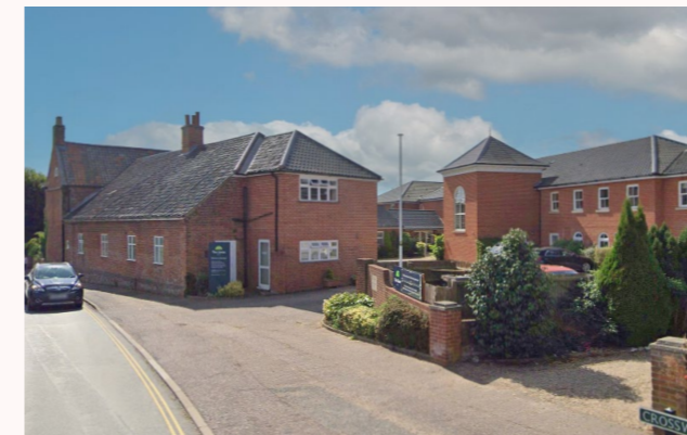
Figure 123: The Limes is a retirement centre of apartments that is converted from a C18th L-shaped building block.
