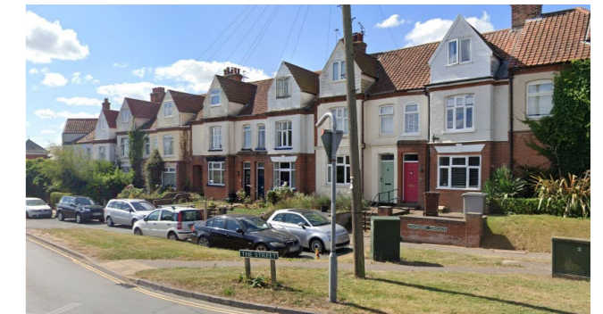
Figure 65: Street parking behind a green verge at Crossway Terrace which could be combined with landscaped screening.
