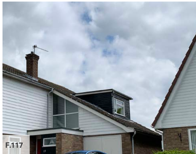
Figure 117: Ill-placed and out of proportion shed dormer, elsewhere in the UK
