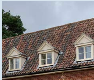
Gabled roof dormer
