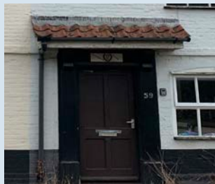
Flat roof porch feature
