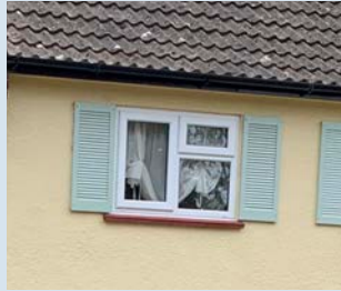
Window with external shutters
