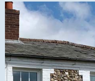
Slate tile roof
