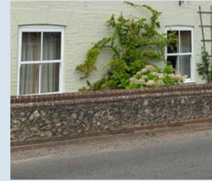
Gault brick wall
