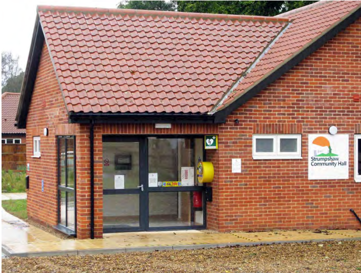
Figure 48: Strumpshaw Community Hall.
