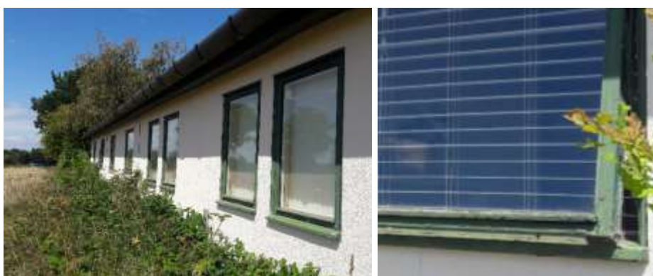
Figure 8: Poorly Fitting Wooden Windows in The Annexe.
