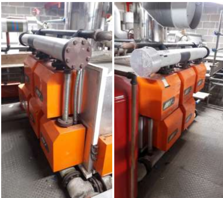
Figure 6: The Pool Natural Gas Heating System
