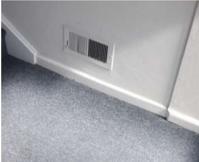
Figure 2: Cavity Air Vent Located at the Foot of the Staircase in the Hall
