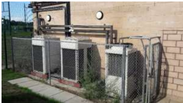
Figure 4: HVAC Condenser Units Supplying Space Heating
