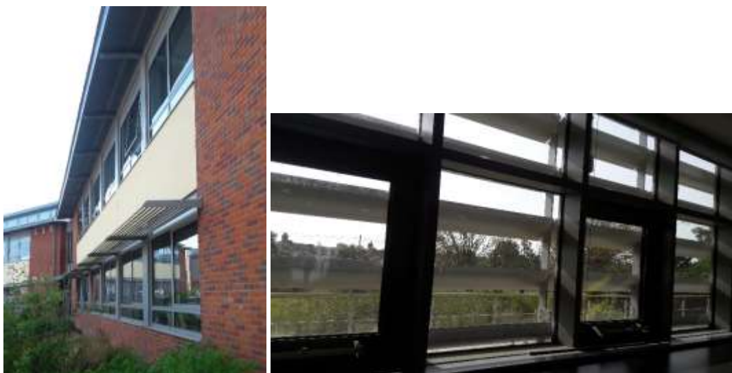
Figure 4: Solar Shades and Over Hanging Roof Reduces Solar Gain.
