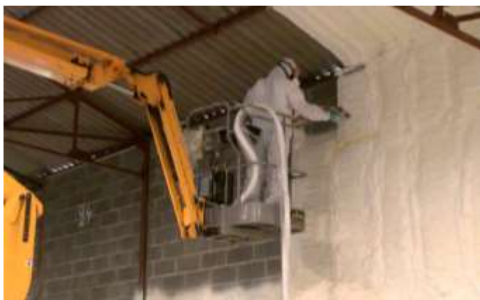
Figure 8: Spray Insulation
