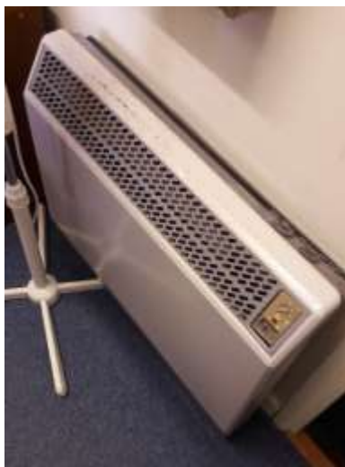
Figure 9: Storage Heater in the Reception Office.
