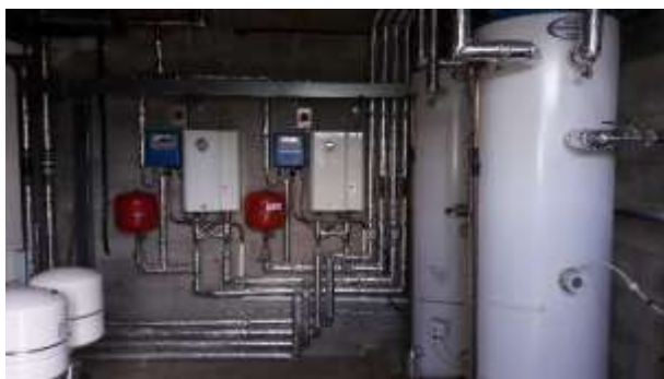
Figure 5: Twin Calorifiers and Water Storage Vessels
